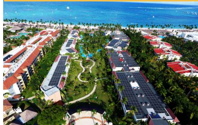
1,2 MWp, Dominican Republic, 2016 Client: AE Co
